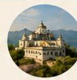
Sajjangarh (Monsoon Palace)
